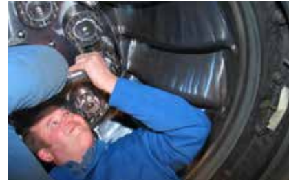
With Superbolt tensioners, joints in awkward positions in confined spaces can be tightened. This Francis wheel has regular maintenance requirements which became manageable with MJTs connecting the wheel to the shaft.
