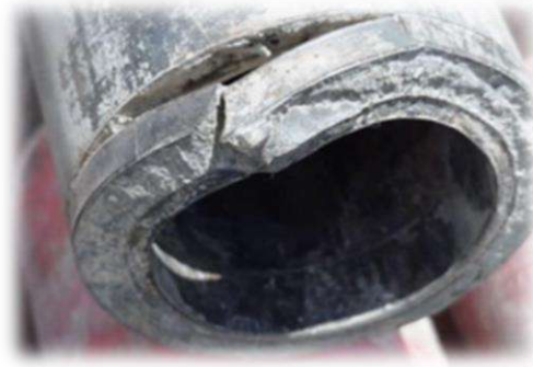
Sour Corrosion ( H 2 S Corrosion)
