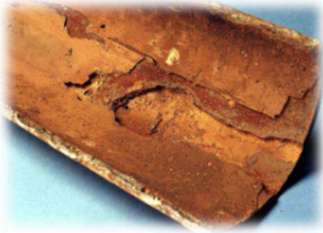
Sweet Corrosion ( CO 2 Corrosion)
